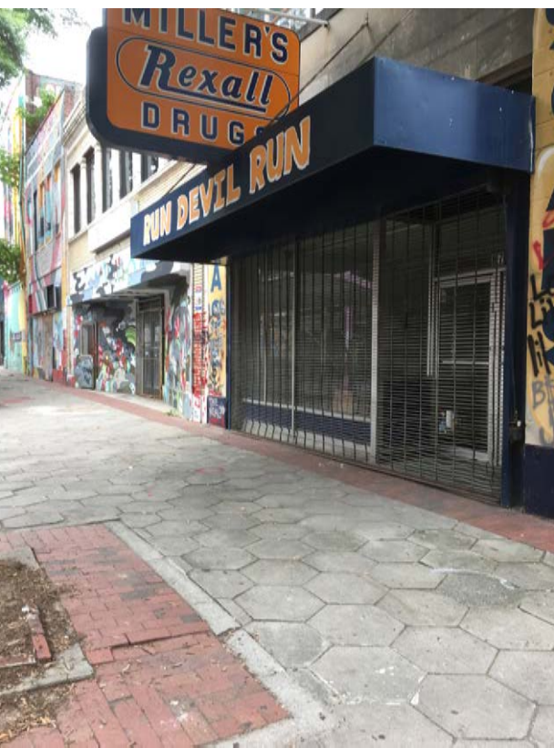
EXISTING LOCATION STOREFRONT
